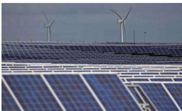
Kamuthi solar power plant
