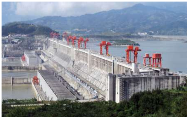
Three Gorges Dam, China
